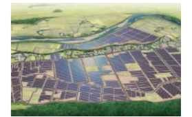
Mega Solar Power Plant in the Yatsuda District of Namie Town, Fukushima Prefecture
