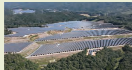
Omuro Mega Solar Power Plant (Agano Mega Solar GK*) * This limited liability company was jointly founded by Mitsubishi Research Institute, Inc., Tokyo Century Corporation, Kyocera Corporation, Rexport, Ltd., and Yonden Engineering Co., Inc.
